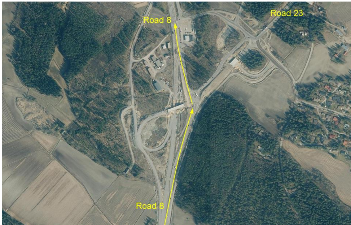
Figure 15: Interchange of the road 8 and road 23 is under construction.
